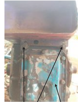
Tank securing bolts
