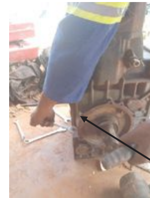
Enlarging gap using spanners
