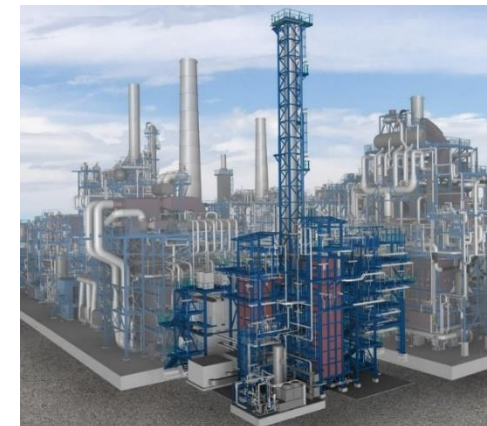
3D graphic of world's first demonstration plant for large scale electrically heated steam cracker furnaces integrated within existing facility
